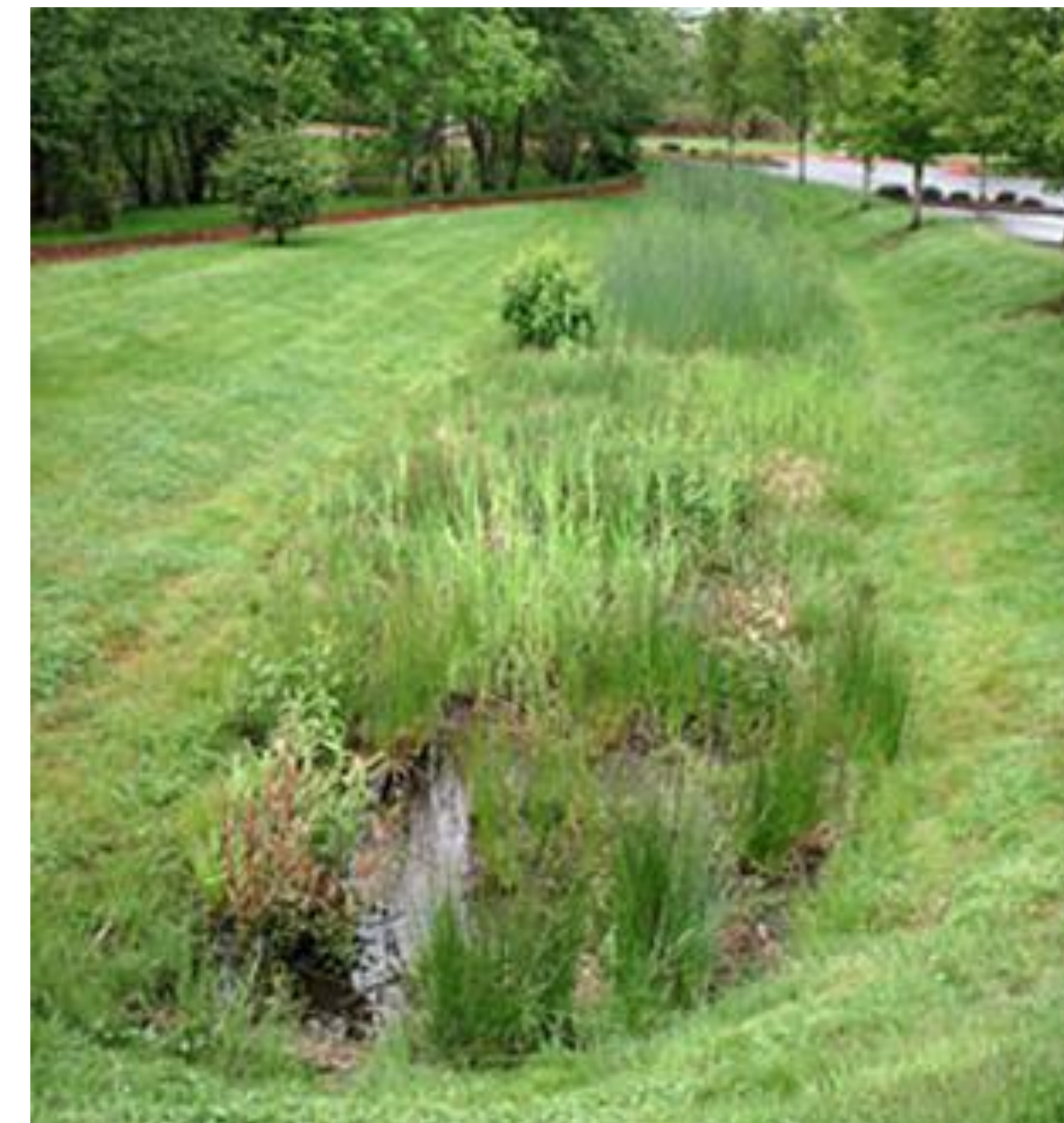
(Example detention basin image)
